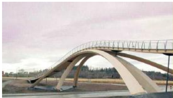
Figure 2: Leonardo Bridge, Aas, Norway.
