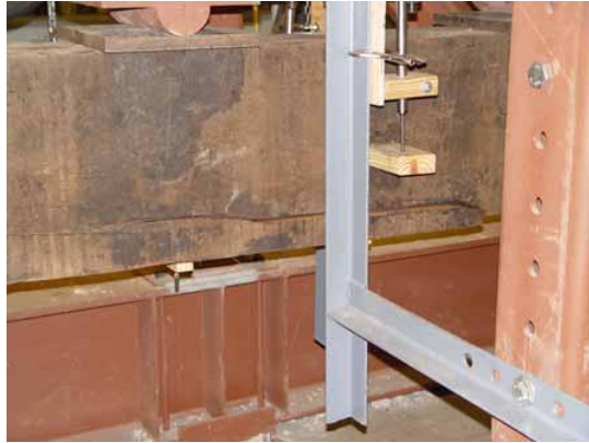
Figure 7: A cross grain tension crack (1).
